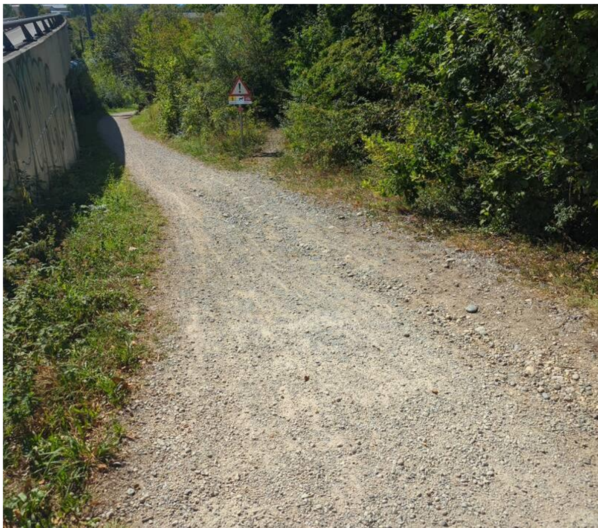
Badly rideable cycle and pedestrian path between Augarten and Kaiseraugust. The steep gradient and loose gravel make it difficult to cycle on a regular touring bike.
