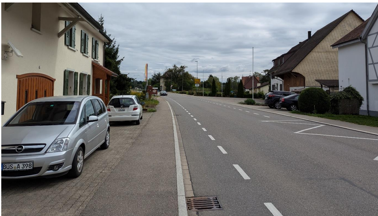
Painted cycle lane. For ECS purposes, this was treated as cycling in mixed-use traffic, as the cycle lane does not reach the minimum effective width.
