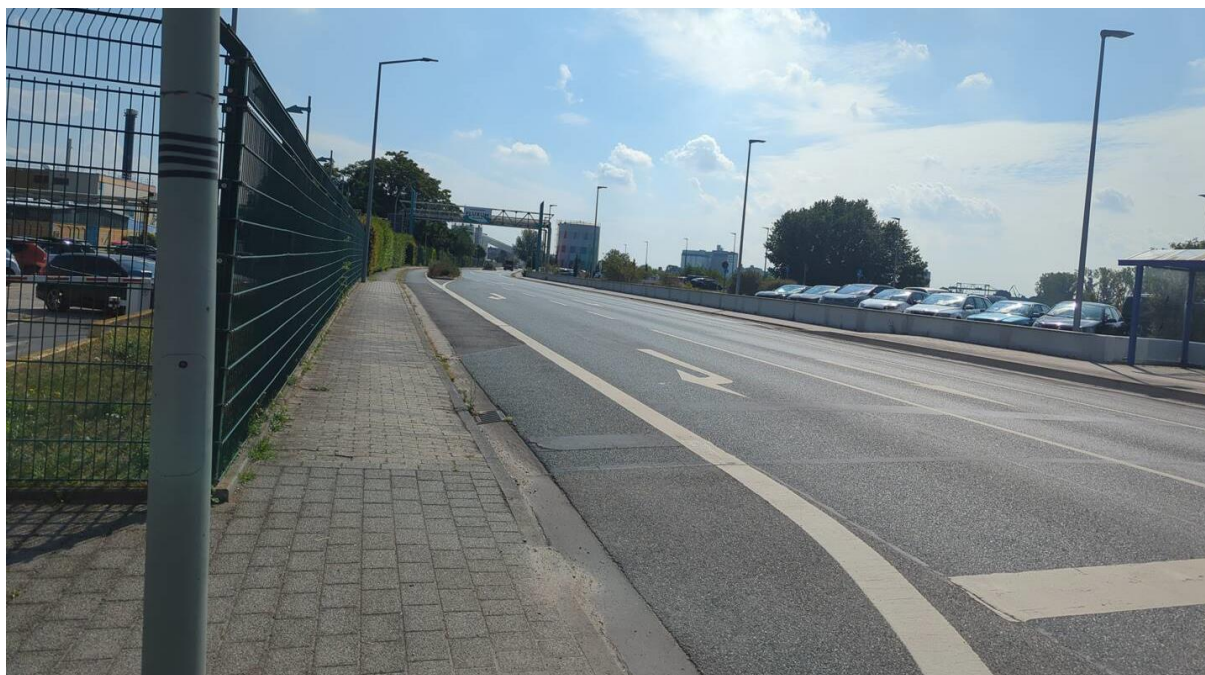
Painted cycle lane. For ECS purposes, this was treated as cycling in mixed-use traffic, as the cycle lane does not reach the minimum effective width.
