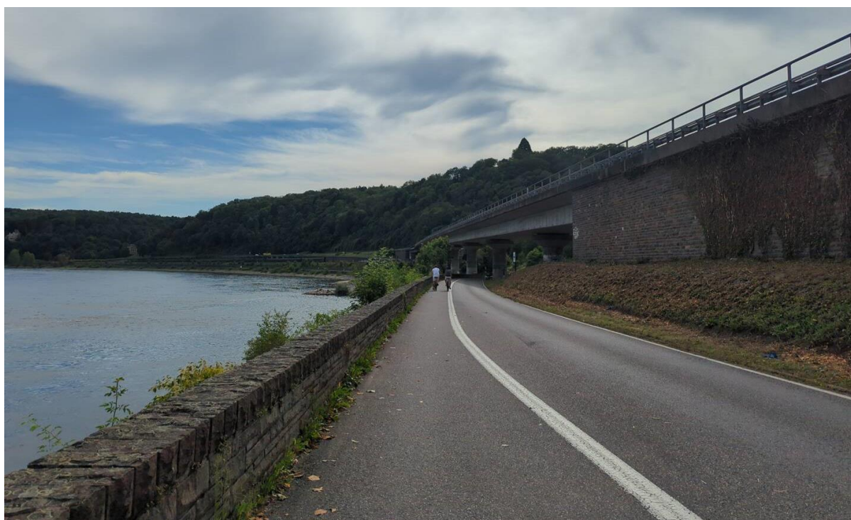
Painted cycle lane. For ECS purposes, this was treated as cycling in mixed traffic, as the cycle lane does not reach the minimum effective width.
