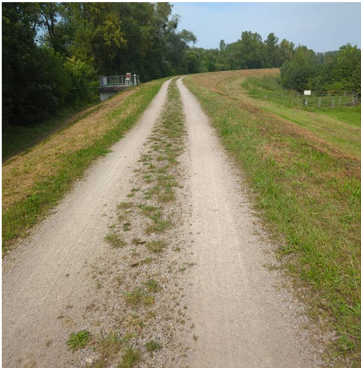
Moderately rideable water management road made from stabilised gravel.
