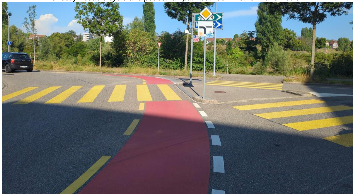
Perfectly rideable painted cycle lane in Basel. For ECS purposes, this was treated as cycling in mixed traffic, as the cycle lane does not reach the minimum effective width.
